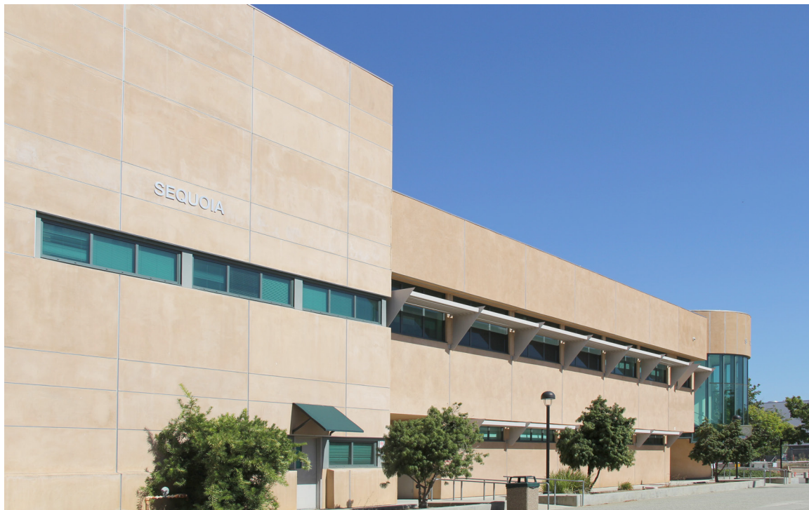
Evergreen Valley College, Sequoia Classroom Building
